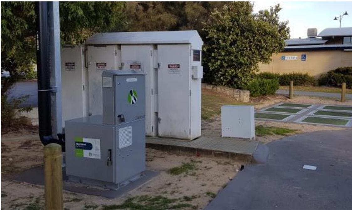
*Figure 2 - Control cubicle, fan cabinet and short (3m) vent stack located with existing pump station switchboard, and biofilter units in background.*
