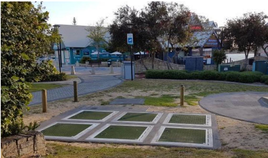
*Figure 1 - OdaVent MHV Biofilters concealed under easy-lift covers, with pedestrian footpaths and restaurants in the background.*
